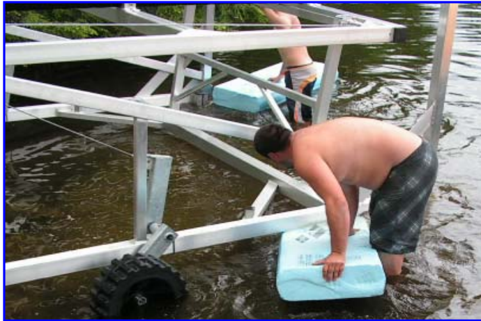
3 Loosen top & bottom leg adjustment bolts
