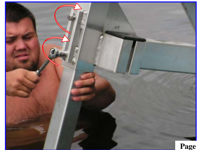
5 Tighten top & bottom leg adjustment bolts
