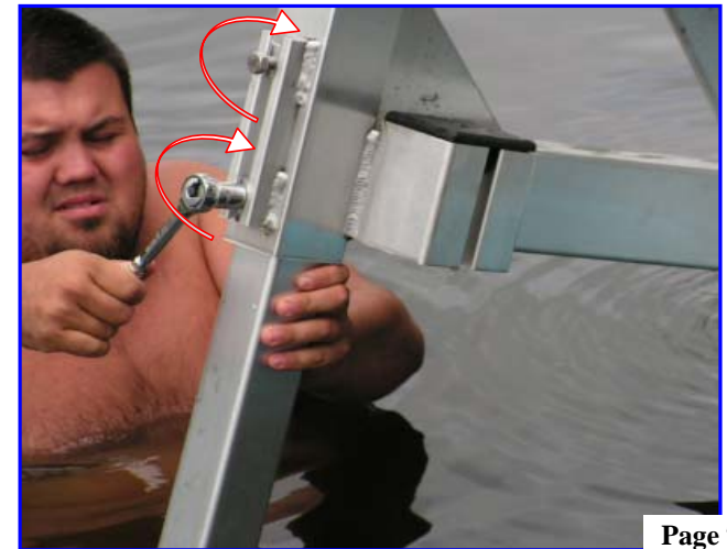
5 Tighten top & bottom leg adjustment bolts
